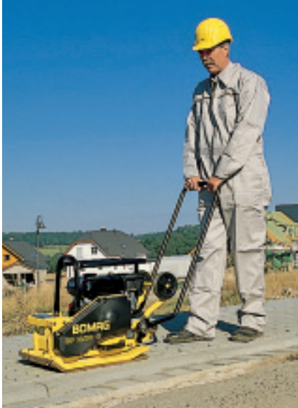
Compacting paving blocks with vulcolan mat
